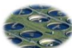
Waste Water Management
